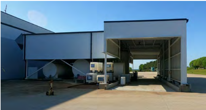
Our Huntsville, Alabama, facility implemented an improvement project that significantly minimized generation of industrial wastewater and stormwater. The improvements included wastewater evaporation technology and enclosure structures for a storage tank area and loading dock ramps. The evaporator reduces the volume of wastewater, whereas enclosures eliminate stormwater runoff flowing into the facility’s industrial wastewater collection system. The project resulted in an annual 99.3% reduction in the amount of wastewater disposed and 97.2% of cost saving for waste hauling and disposal.
