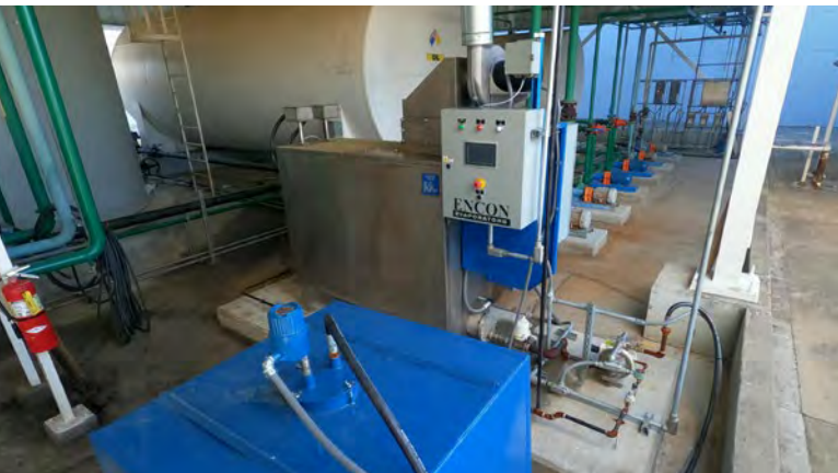
Our Huntsville, Alabama, facility implemented an improvement project that significantly minimized generation of industrial wastewater and stormwater. The improvements included wastewater evaporation technology and enclosure structures for a storage tank area and loading dock ramps. The evaporator reduces the volume of wastewater, whereas enclosures eliminate stormwater runoff flowing into the facility’s industrial wastewater collection system. The project resulted in an annual 99.3% reduction in the amount of wastewater disposed and 97.2% of cost saving for waste hauling and disposal.
